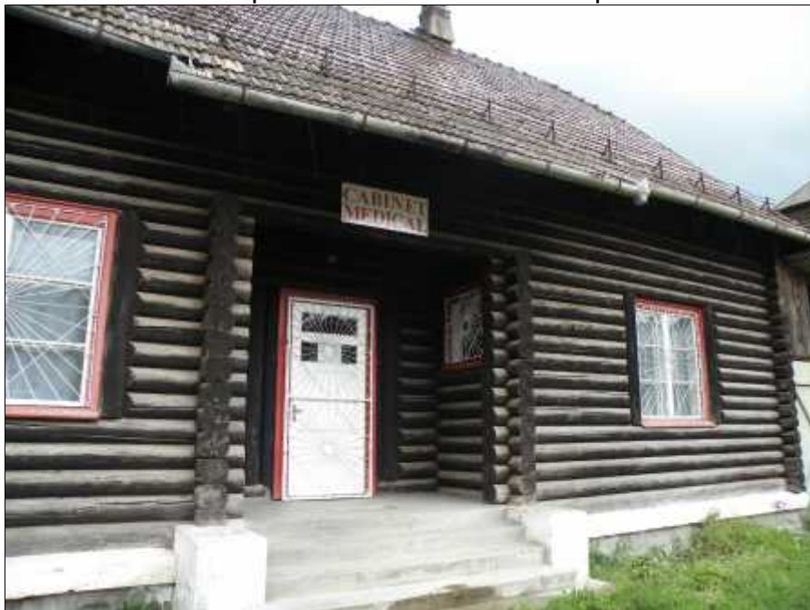
Img. 13 – Cabinet medical – amplasament provizoriu
