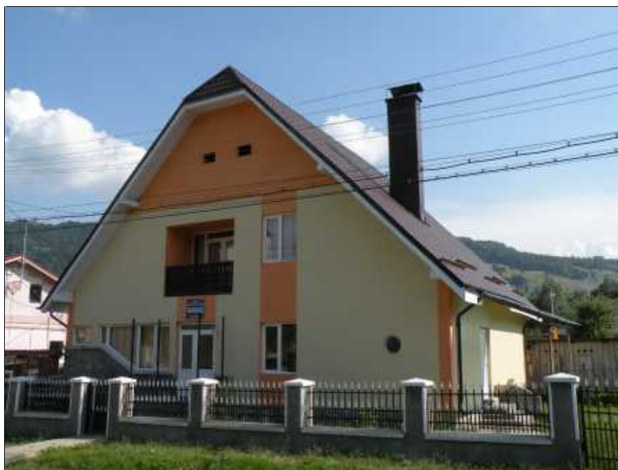
Img. 5 – Gradinita sat Bicazu Ardelean
